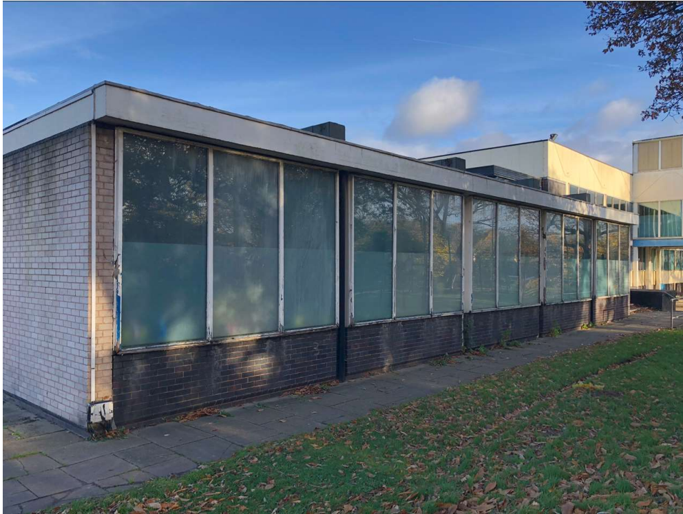
Photo 3: Southwest elevation, Teaching Pool. The timber framed windows are rotten and require replacement.
