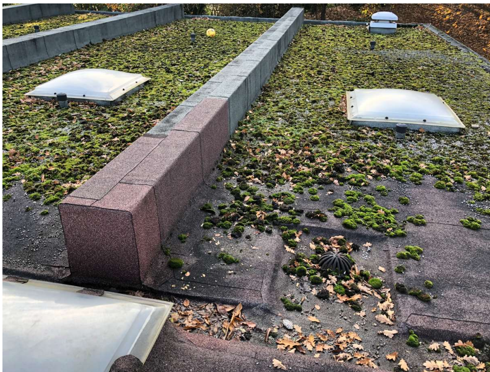
Photo 40: Roof over Teaching Pool. Beams project above.
