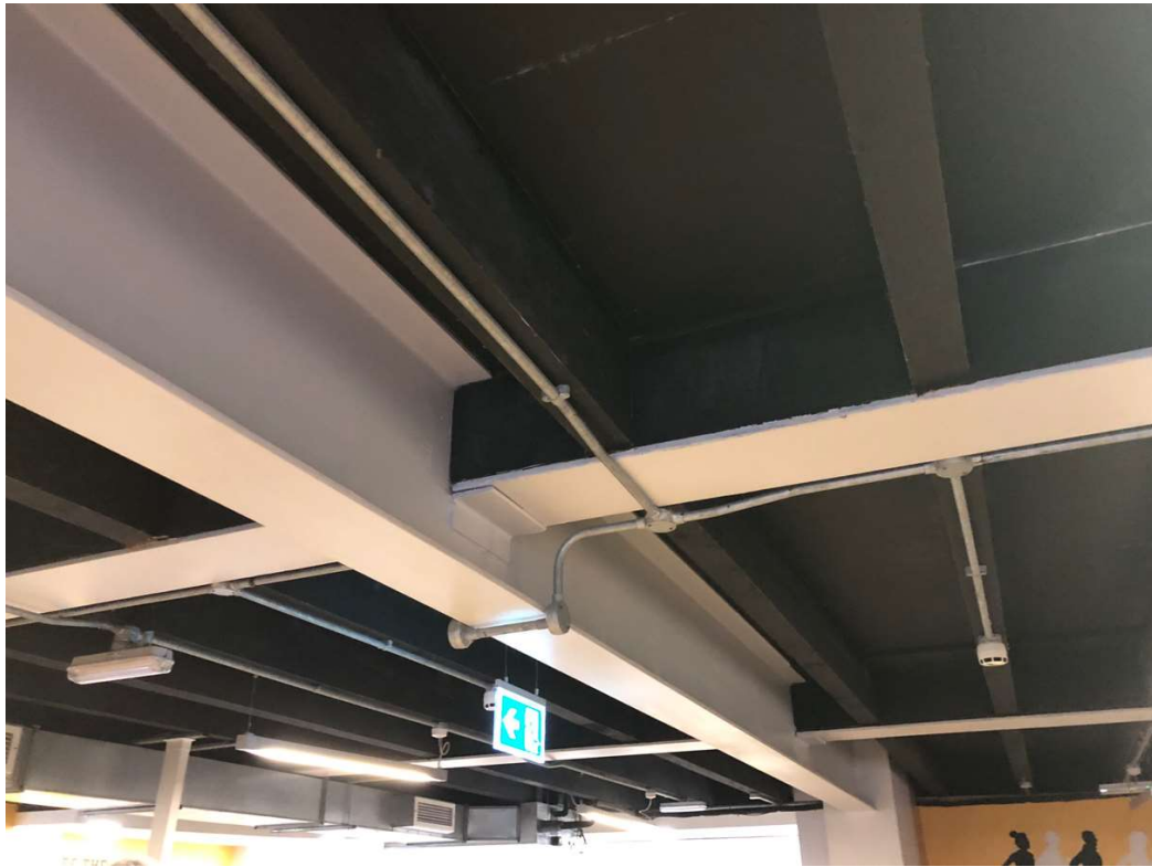
Photo 44: Underside of first floor structure.
