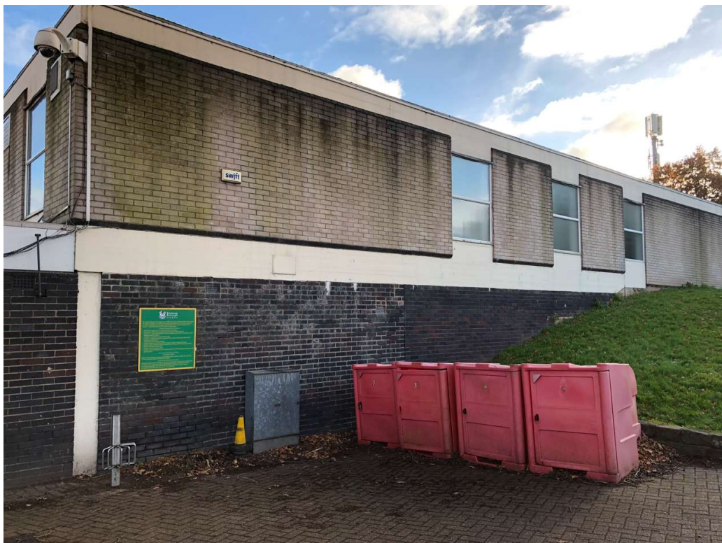
Photo 2: Northwest elevation. Brickwork in reasonable condition.
