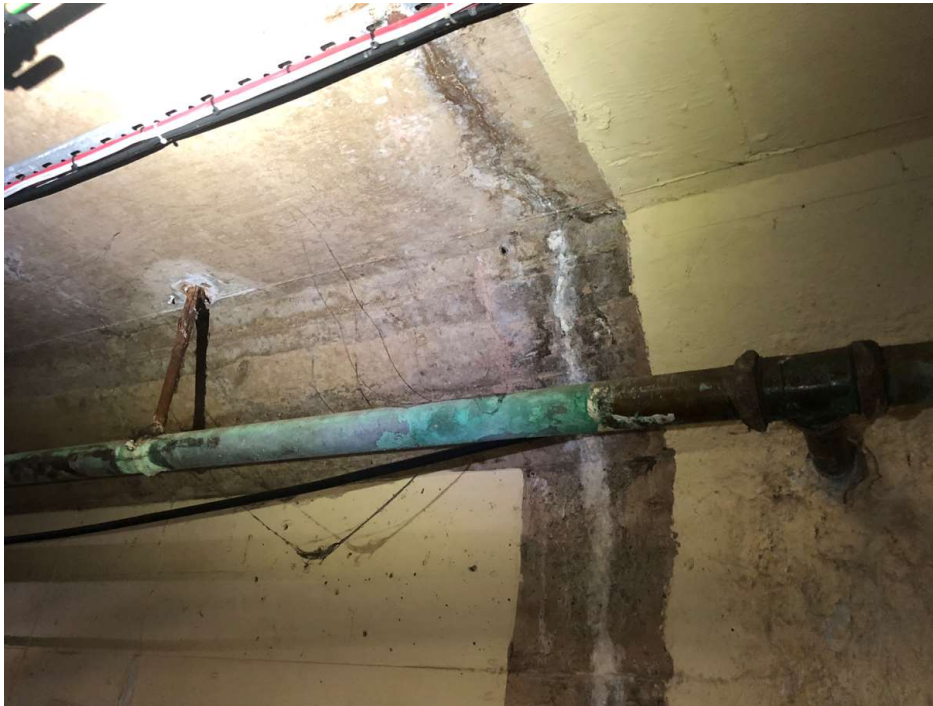
Photo 31: Main Swimming Pool tank. Vertical cracks are present in the walls. These are not considered structurally significant but should be surveyed annually to check their severity does not change.
