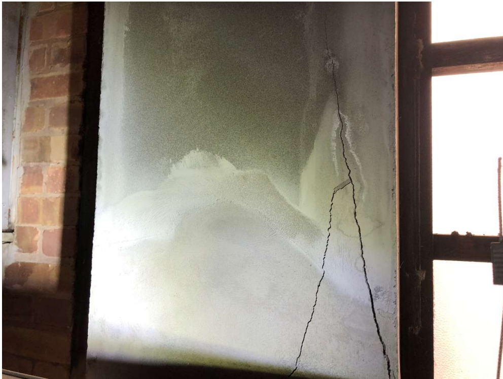
Photo 23: Pool basement column repaired with high strength mortar, but the repair has partially failed.
