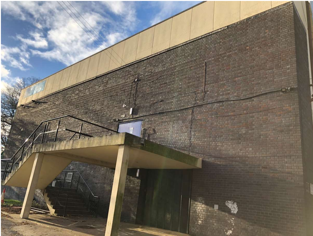
Photo 9: South elevation. Concrete escape stairs from Main Pool.
