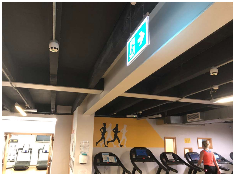
Photo 44: Internal view within the converted squash courts. The steel beam is supporting the remainder of the loadbearing masonry wall above. The floor is timber joisted.
