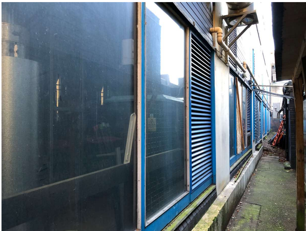
Photo 10: Southeast elevation of Main Pool at basement level.
